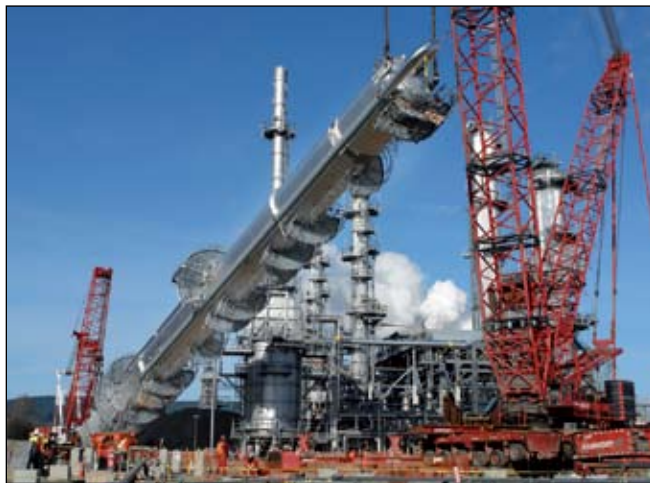
Largest column being set on foundation. Inset (right): John Brentari, Project Mgr, Shell; Steve Nelson, Staff Project Engineer, Shell; Steve Dahl, Project Mgr, J.H. Kelly LLC.; Paul Morton, Construction Mgr., DH2MHill Inc.
