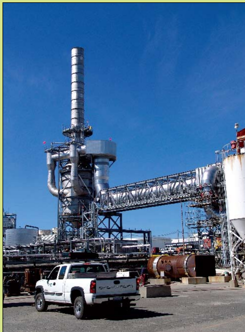
Shell Puget Sound Refinery's new Wet Gas Scrubber.
